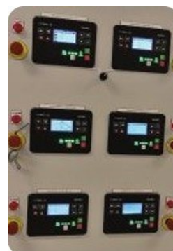
Generator synchronising
